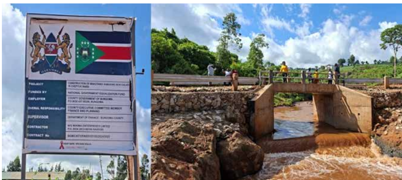
Picture 8: Makutano-Kabukwo box culvert in Bungoma County
