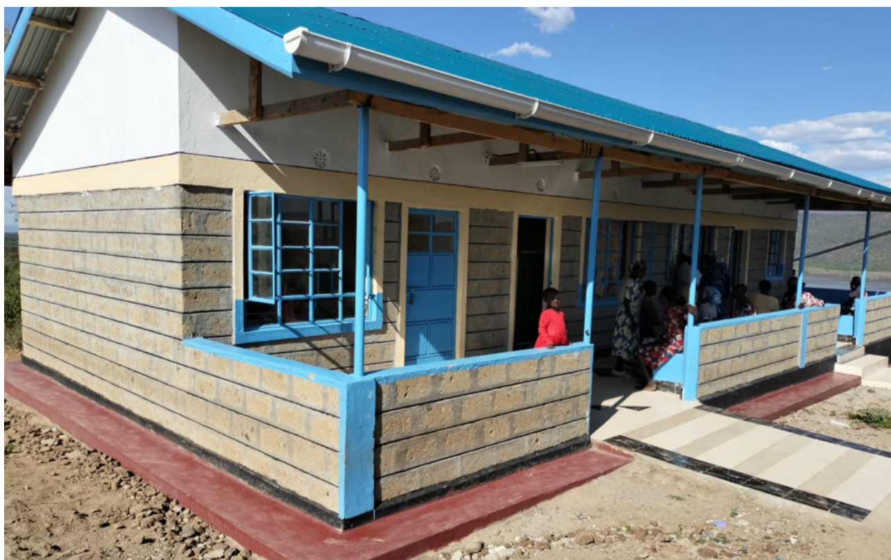
Picture 11: Newly constructed Lobo Dispensary, Mochogoi Ward, Baringo County. Construction of Kataboi Eco Lodges
