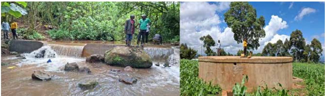
Picture 6: Water Intake (left) and distribution tank for the Sambocho Water project
