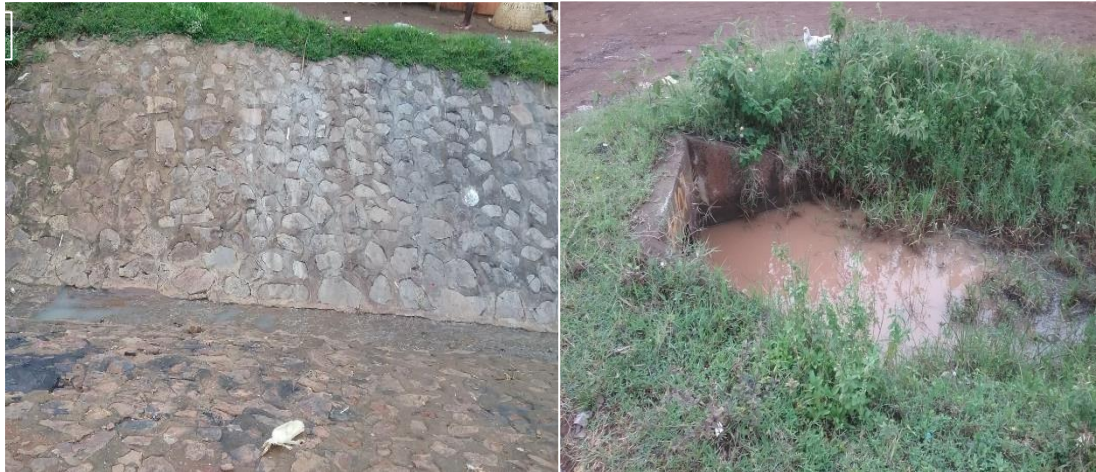
A Paved Storm Water Drainage Channel
