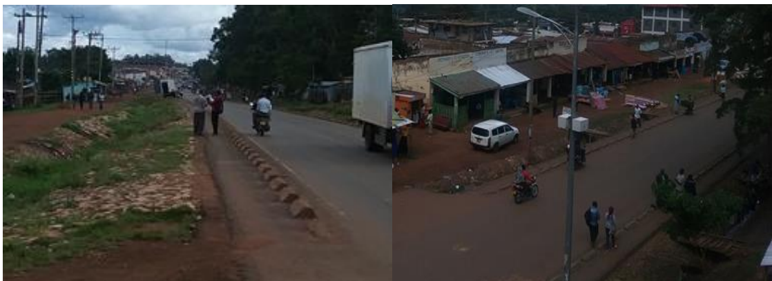
Existing Condition of Pedestrian Walkways
