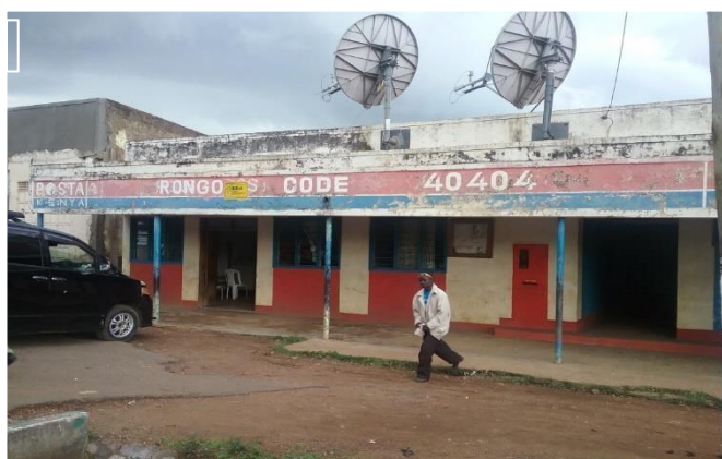
Figure 39: Rongo Post office
