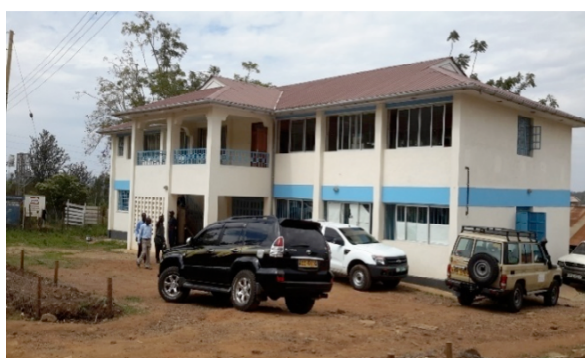
Administration/Drugs Store Block Constructed At Migori County Referral Hospital
