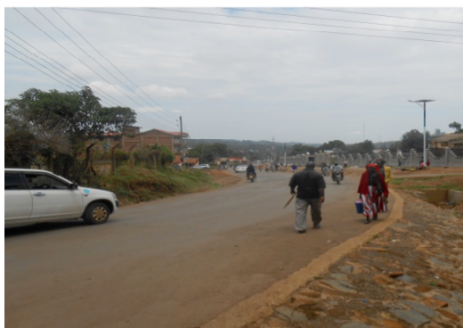
Posta – Ombo Ring-Road after Completion
