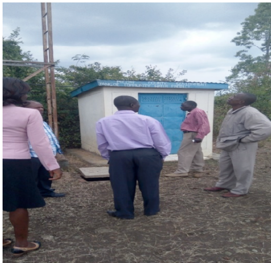
Jangoye water supply system
