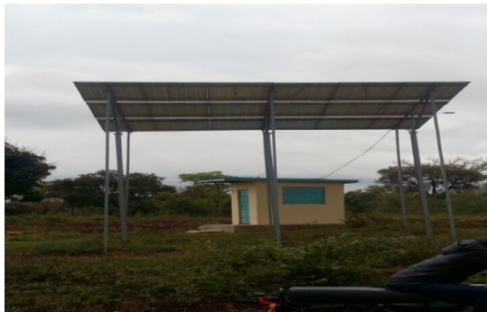
Mukuro water project supply system
