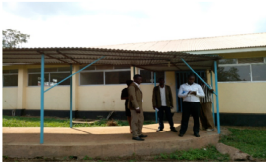
Mortuary at Kehancha Dispensary
