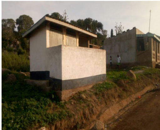
Toilets constructed at Nyangwina Landing site
