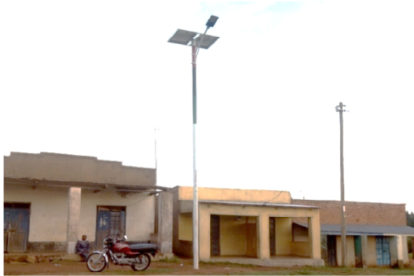
Giribe solar lighting project in wasimbete ward
