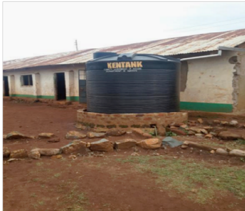
Siling primary water tank in Suna East Sub-county
