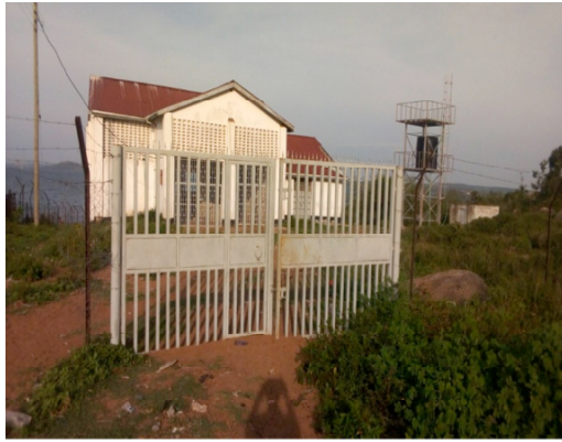
Completed Nyangwina landing site in Muhuru Bay ward
