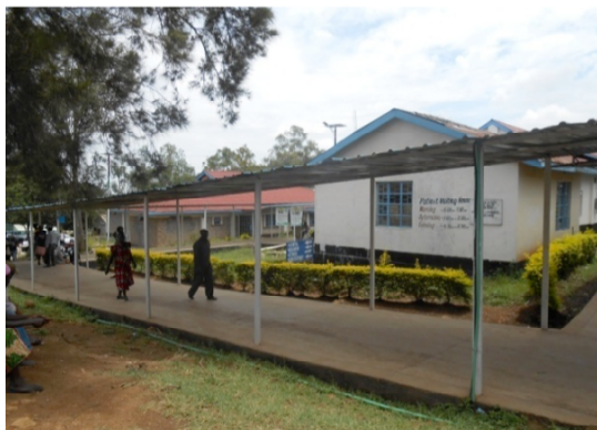
Renovated Migori Phase II Level IV Hospital
