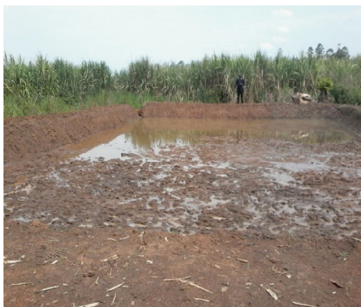
Fish pond under construction in Awendo
